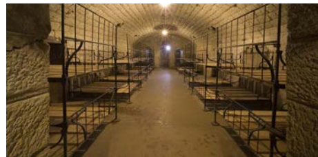
Casemate for the barracks at Fort Douaumont © Jean-Luc Kaluzko
